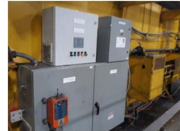
Wireless remote I/O on cranes
